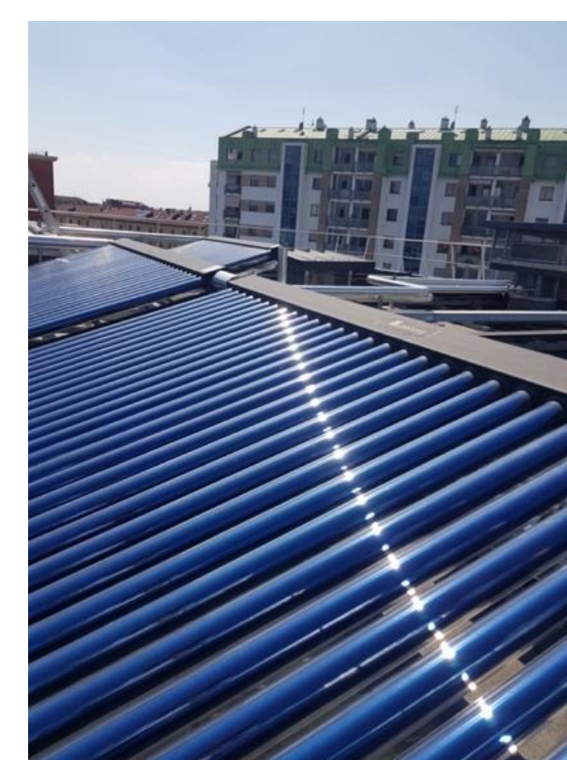
Fig. 6: Solar vacuum tubes on the building's roof.
