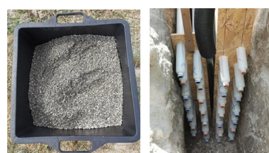
Fig. 9: Sand mixed with granules with paraffin and cylindrical high-density polyethylene containers filled with hydrated salts (Bottarelli et al., 2022).
