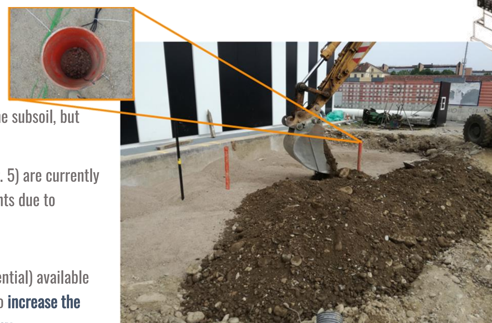
Fig. 5: Plastic pipes introduced before final ground backfilling in 2019 during the installation of very shallow sensors.
