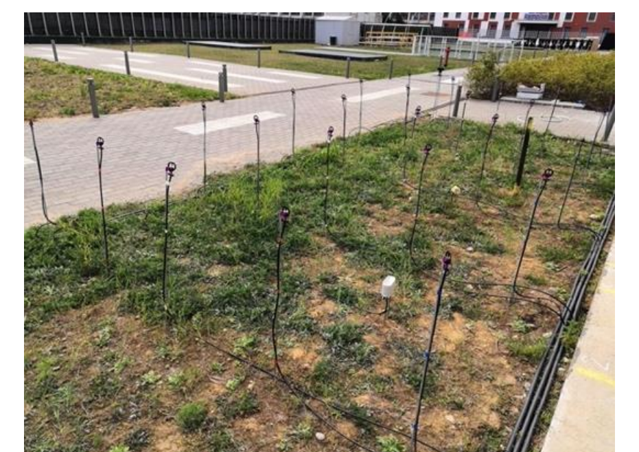
Fig. 3: Sprinklers system installed in the shallow layers of the ground.
