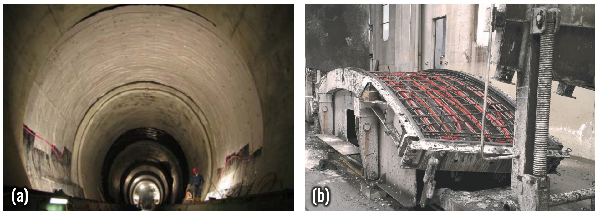
Fig. 3 – Instrumentation of (a) conventional and (b) mechanised tunnels of heat exchange.
